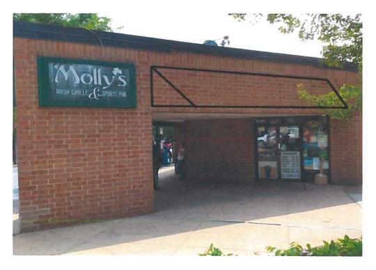
**1.Install new awning above opening at 8**4<sup>th</sup> Street rear. Awning to be the same configuration as 4<sup>th</sup> Street elevation (There was an awning at this elevation at some point as fasteners are still on building). Awning fabric to match 4<sup>th</sup> street awning.
